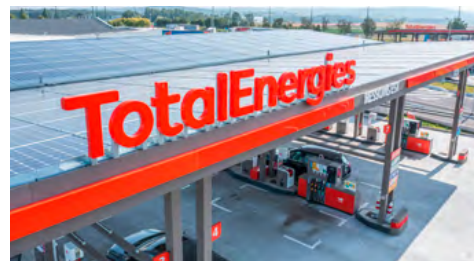
Solar panels on the roof of a service station in Ressons (France).
