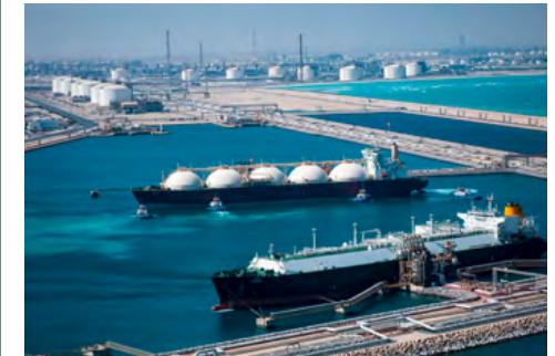
Ras Laffan liquefaction terminal Doha (Qatar).
