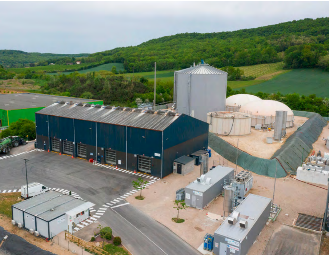
The BioVilleneuveois methanization plant in Villeneuve-Sur-Lot (France).
