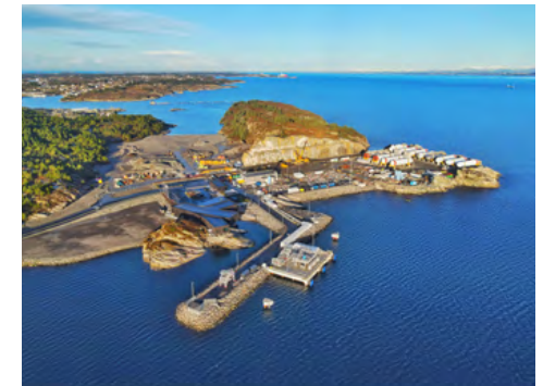
The Northern Lights CO 2 receiving, storage and pumping terminal, now under construction in Øygarden, (Norway).
