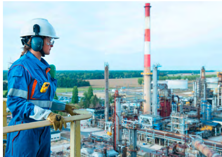
Operator at the Grandpuits zero crude platform.
