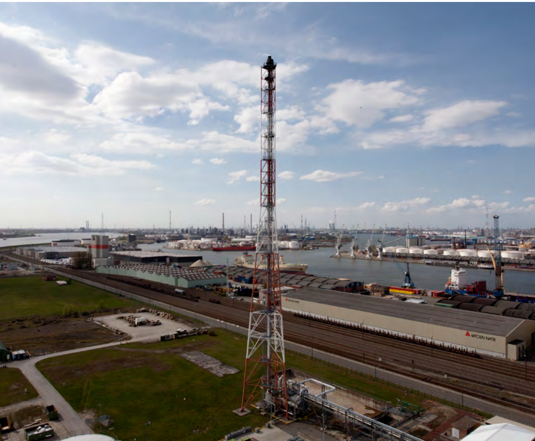
Antwerp refinery (Belgium).
