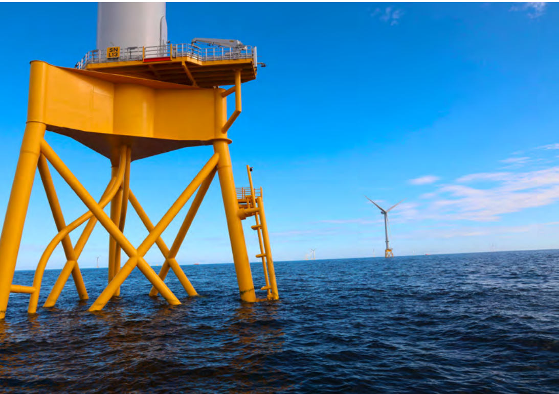
Seagreen (Scotland) offshore wind farm under construction.
