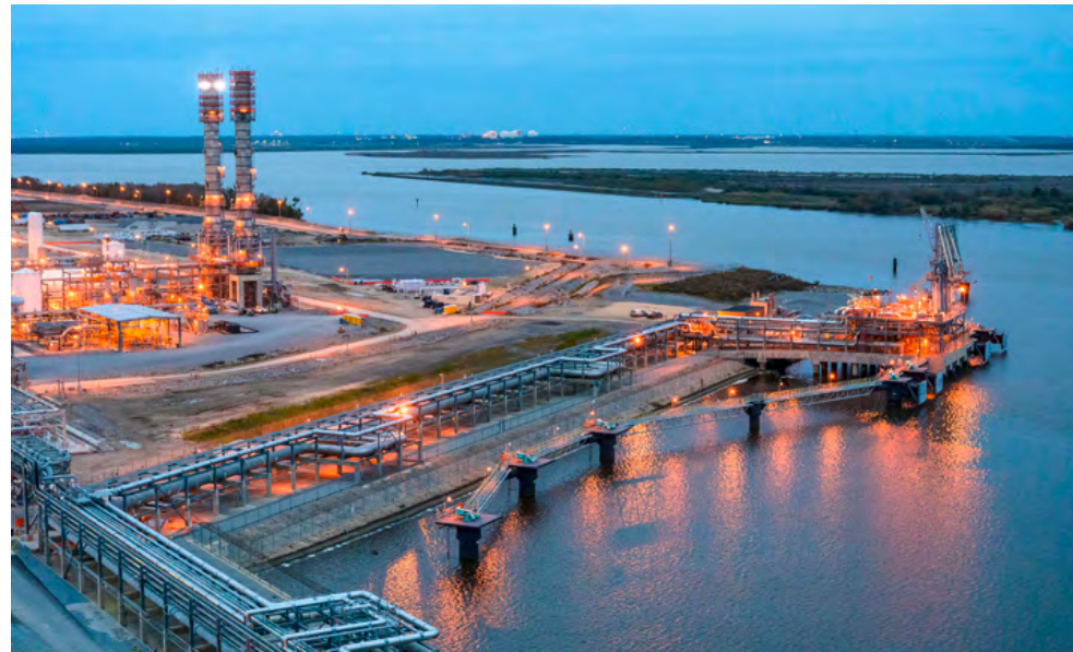
Cameron LNG liquefaction terminal, next to Lake Charles, Louisiana, USA.
